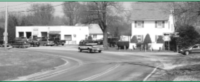
The three-way intersection of Route 82 and Doe Run Road will soon be converted to a one-lane roundabout.
